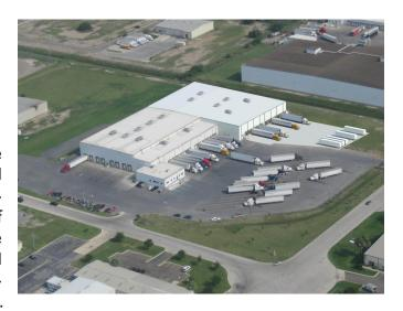
Primus was challenged with providing a flexible floorplan to handle extremely high storage and retrieval volumes and an ever-changing product mix. During peak seasons, the facility must be able to handle up to 200 trucks per day. Also, due to Loop's requirement for tight temperature tolerances in the event of compressor failure, the refrigeration system is designed so that any given room will remain at 80% refrigeration capacity.
